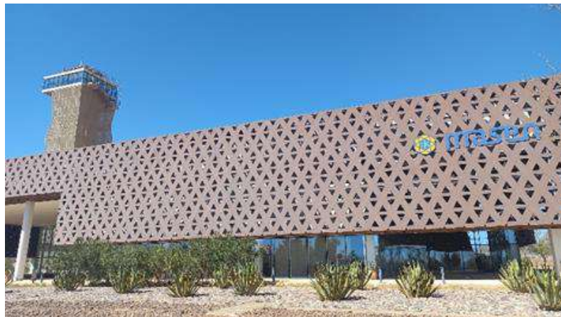
Figure 14 PHIL laboratory building at Masen
