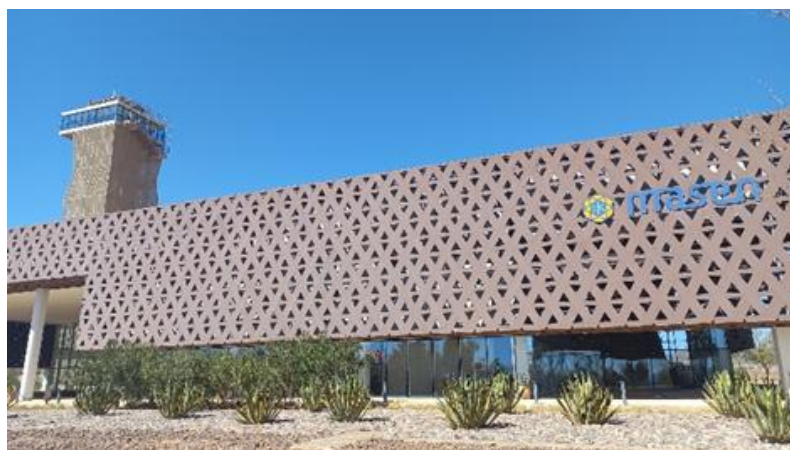
Figure 14. PHIL laboratory building at Masen
